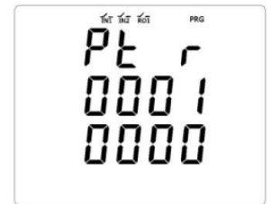
Potential Transformer Ratio
